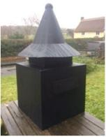
on top. The two vents are covered inside with mesh to allow for ventilation whilst preventing access to unwanted nest-builders.
